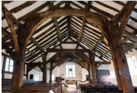
Interior of Old Church
